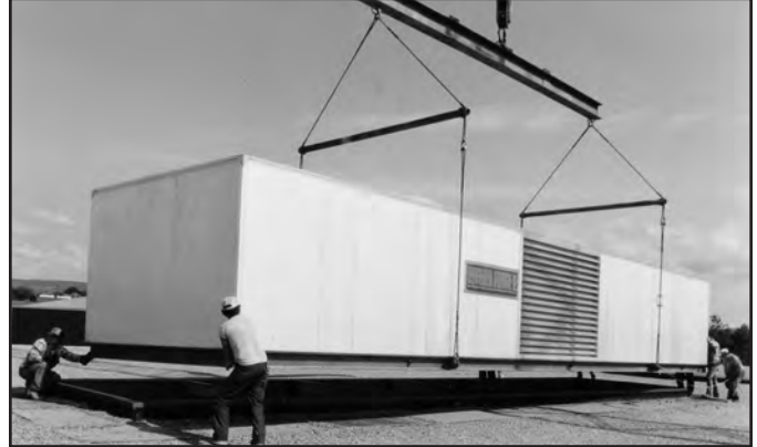
Units are completely fabricated and pre-assembled at the factory to ensure proper fit when joined in the field. These units are shipped in large modules requiring the least amount of field assembly and installation time.
